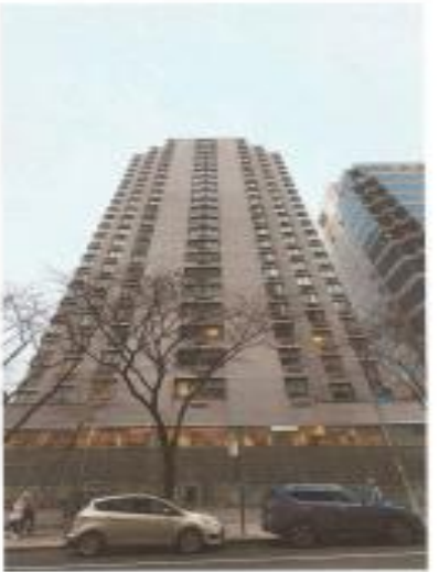
3. VIEW LOOKING SOUTHWEST
